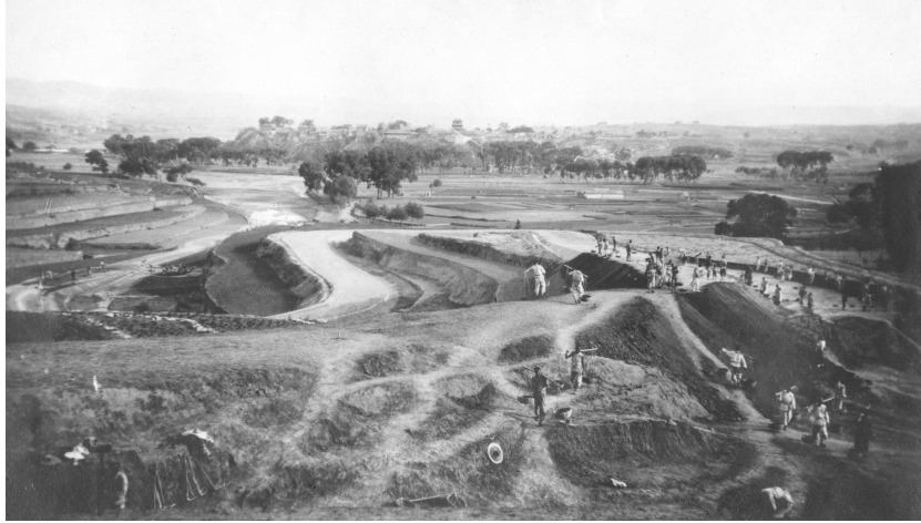
Finishing work on the road north of Xiyang.[1]
